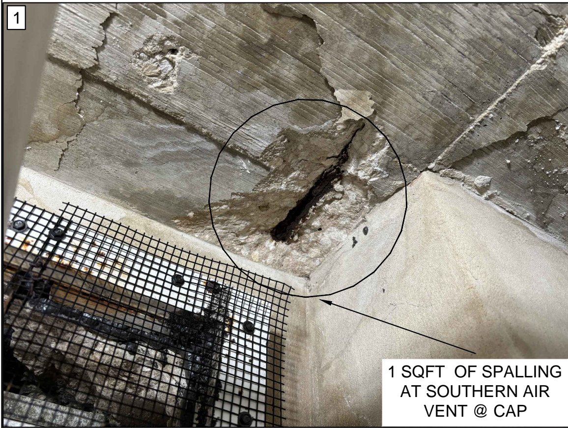
TOP & BOTTOM OF POOL PUMP CONCRETE CAP IS IN GOOD AND SERVICEABLE CONDITION. BOTTOM OF POOL PUMP CAP HAS MINOR SPALLING.
