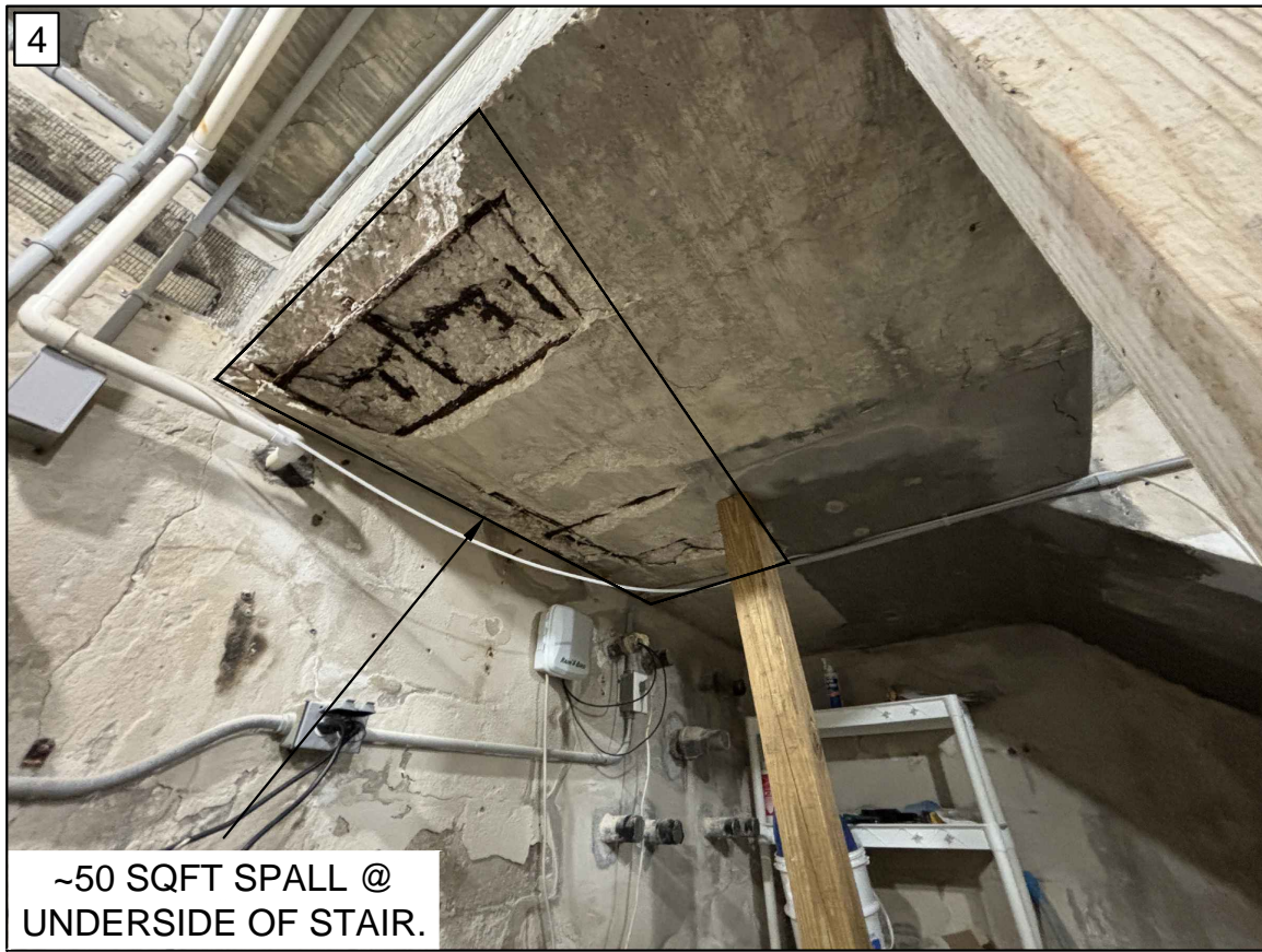
CONCRETE DAMAGES ARE PRIMARILY UNDER THIS STAIR FLIGHT.
