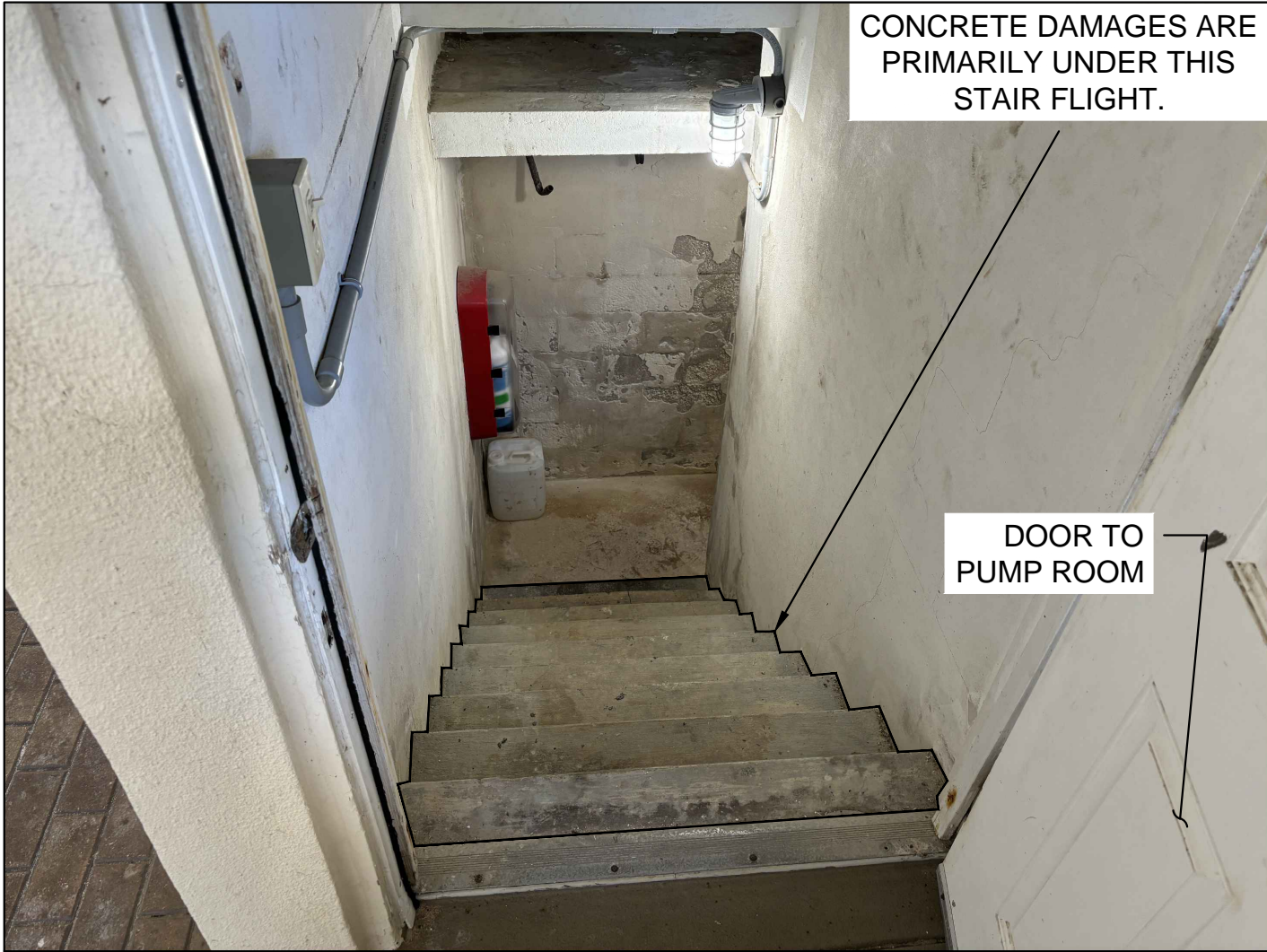
~50 SQFT SPALL @ UNDERSIDE OF STAIR.
